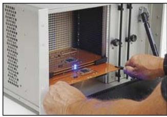
Installing an output expansion switch blade
